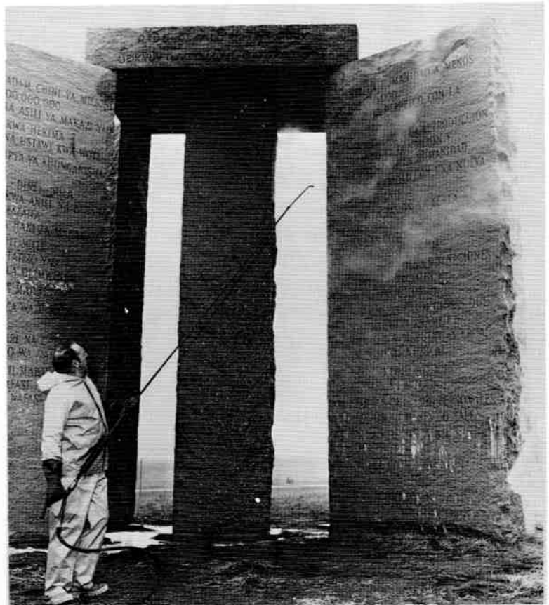
The Georgia Guidestones" get "the final-touch," which is a steam and acid cleaning from Norris Mattox. This brings out the beauty of both the stone and workmanship. Other than this cleaning, the stones and site remain unchanged.
