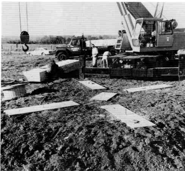
This photo shows the configuration of The Georgia Guidestones® four large outside base slabs, with a central or gnomon stone, arranged like a giant padlewheel with the outer stones oriented to the limits of the migration of the moon during a year. The center stone is marked and holes drilled in it so that the sun rays mark the time of day and the seasons of the year. Also, the North Star is always visible through a special slot from the South to the North side of the center stone. An astronomer was employed to accurately achieve this placement of the stones.
